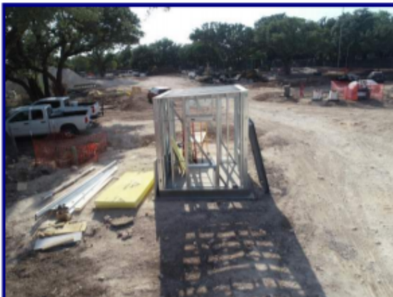
Mock up in progress.
