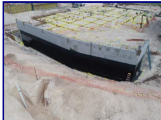
Retaining wall waterproofing in progress.
