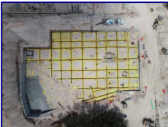
Vapor barrier for level 1 grade beams in progress.
