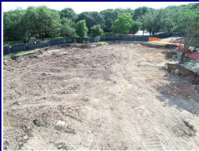
Building demolition substantially complete.
