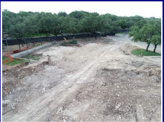
Building demolition substantially complete.
